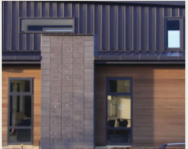
Stack bond masonry block
